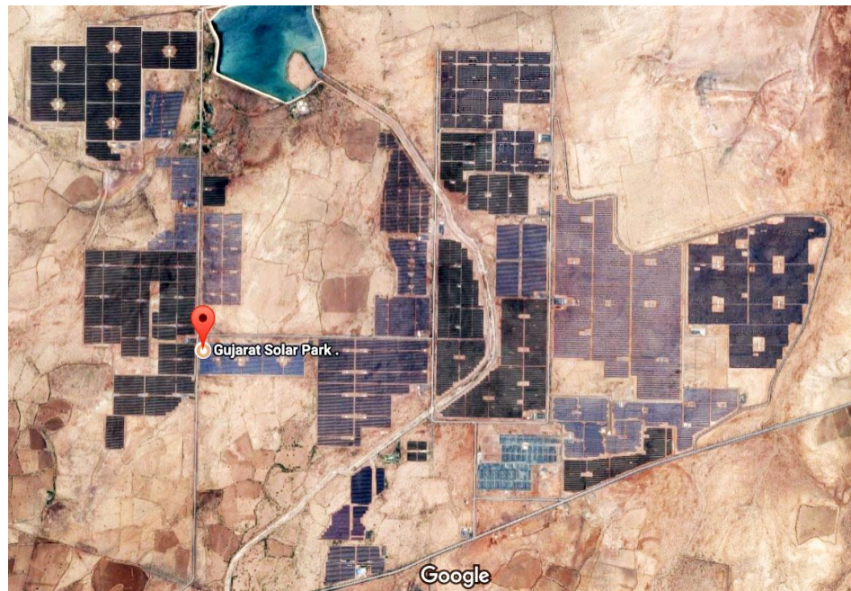
20 MW Solar PV Power Project, Gujarat, India Covering 149 Acres
